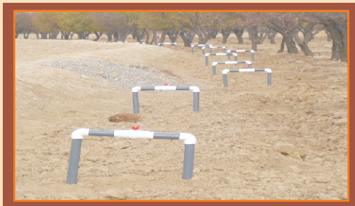
Installation of hydrants for High Efficiency Irrigation System in Loralai
