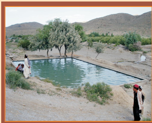
Constructed lined water storage reservoir in Killa Saifullah
